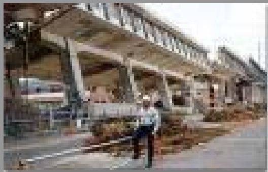
Destroyed Freeway By Earthquake
