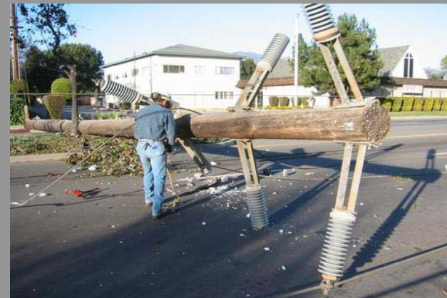
Down Electrical & Phone Lines
